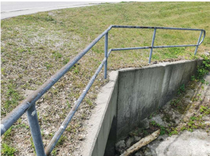
Poor Condition Handrail
